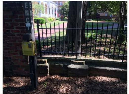
(177), Pendleton Street - Street Elevation Low wall with fence and multiple piers. Transition to large entry pier.
