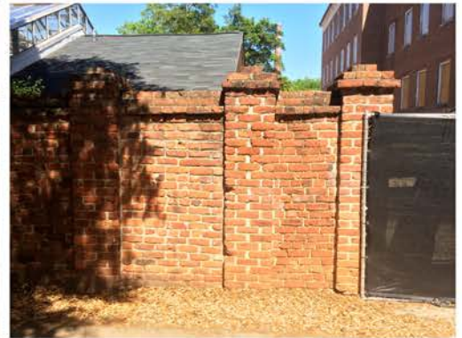
(69), Sumter Street - Street Elevation Full height wall with multiple entry piers. Left side of entry.
