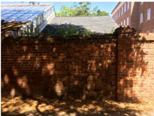
(70), Sumter Street - Street Elevation Full height wall with single pier.
