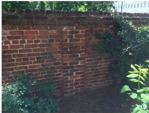
(92), Sumter Street - Campus Elevation Full height wall.
