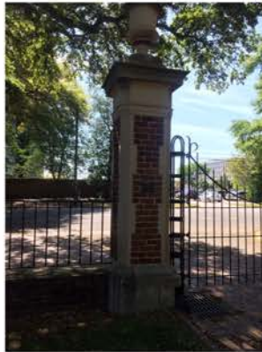
(236), Sumter Street - Campus Elevation Partial height wall with vertical rail to large stone- brick pier.
