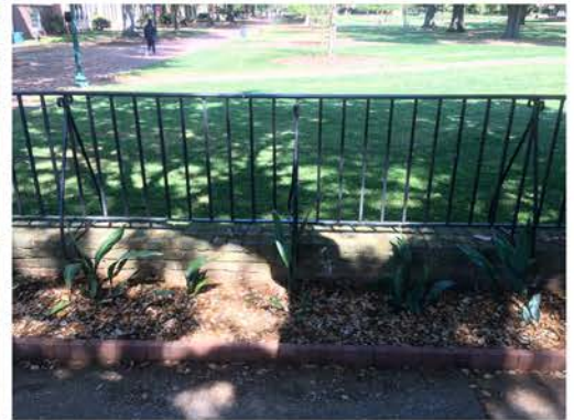
(117), Sumter Street - Street Elevation Partial height wall
