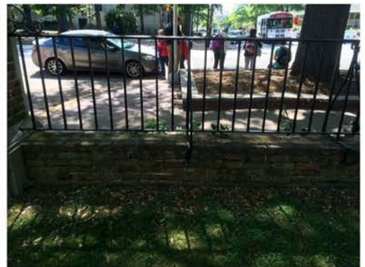
(216), Sumter Street - Campus Elevation Partial height wall with vertical rail.
