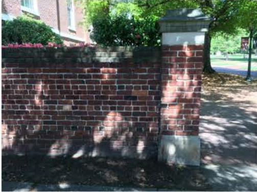
(124), Sumter Street - Street Elevation Full height wall with small pier. Signage.
