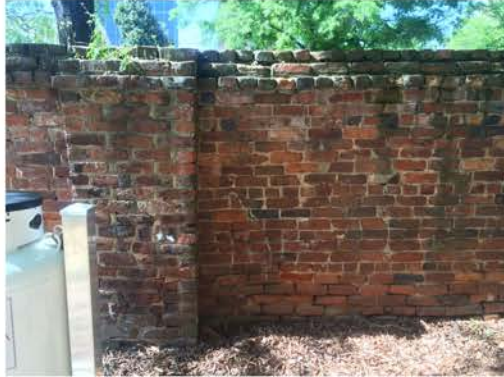
(305), Pendleton Street - Campus Elevation Full wall height. Repointing required. Multiple mortars.
