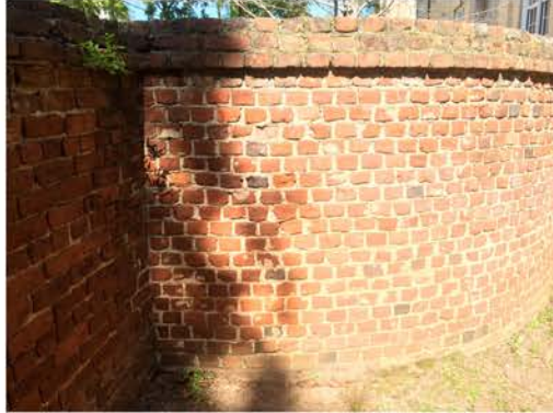
(317), Pendleton Street - Campus Elevation Full height wall curved .
