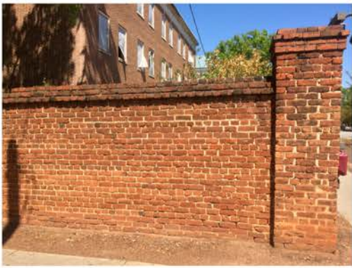
(49), Sumter Street - Street Elevation Full height wall. Corner Pier.
