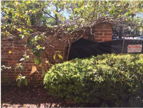
(28), Sumter Street - Campus Elevation Full height wall. Different mortar across wall.
