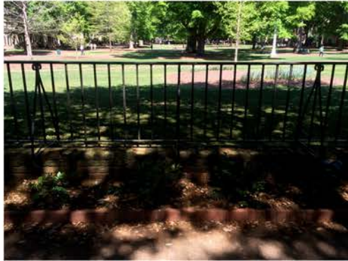
(113), Sumter Street - Street Elevation Partial height wall
