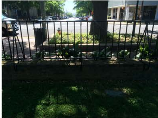
(221), Sumter Street - Campus Elevation Partial height wall with vertical rail. Vegetation issues typ.
