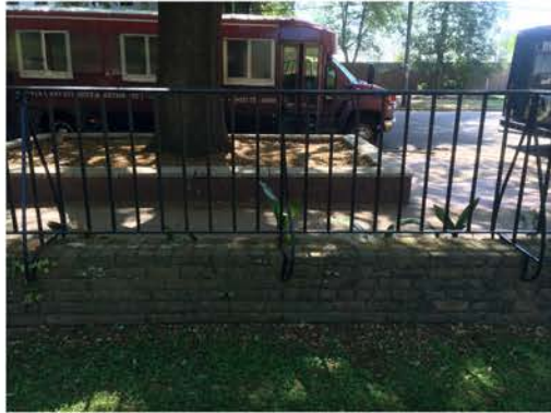
(233), Sumter Street - Campus Elevation Partial height wall with vertical rail. Vegetation issues typ.
