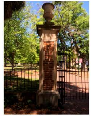
(99), Sumter Street - Street Elevation Large Entry Pier with vertical rail and gate.
