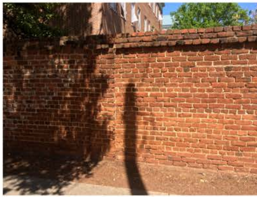
(50), Sumter Street - Street Elevation Full height wall.
