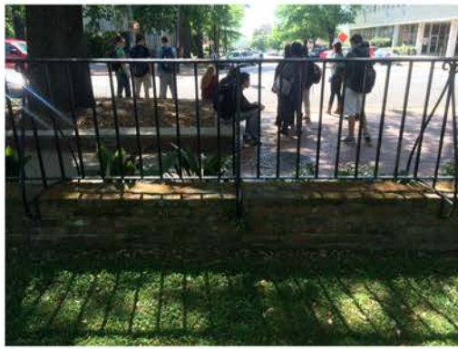
(218), Sumter Street - Campus Elevation Partial height wall with vertical rail.
