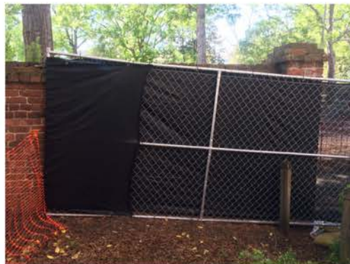
(23), Sumter Street - Campus Elevation Full height wall. New photo required.
