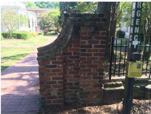
(178), Pendleton Street - Street Elevation Low wall with fence and multiple piers. Transition to large entry pier.
