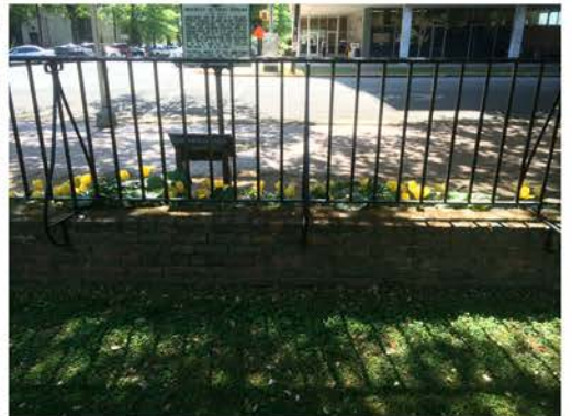
(225), Sumter Street - Campus Elevation Partial height wall with vertical rail. Vegetation issues typ.
