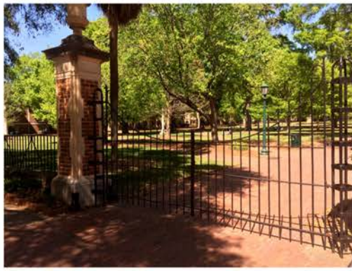
(98), Sumter Street - Street Elevation Large Entry Pier with vertical rail.
