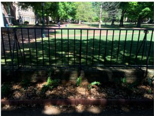
(118), Sumter Street - Street Elevation Partial height wall
