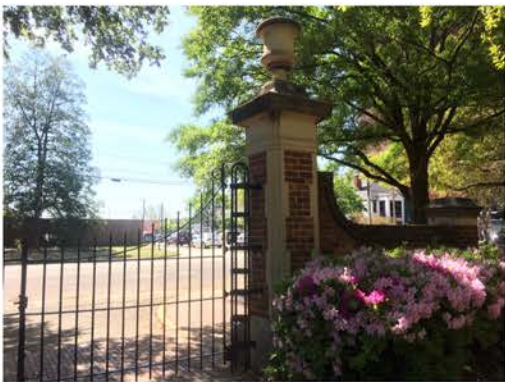
(238), Sumter Street - Campus Elevation Full height wall with vertical rail to large stone brick pier. Gate.
