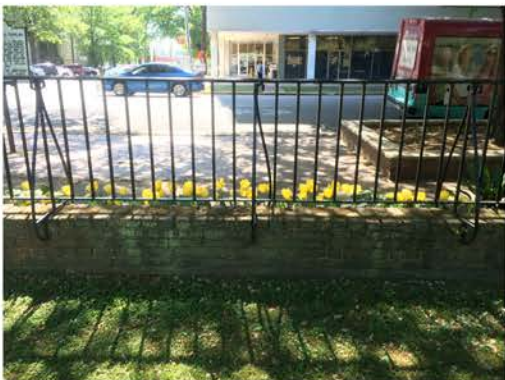
(226), Sumter Street - Campus Elevation Partial height wall with vertical rail. Vegetation issues typ.
