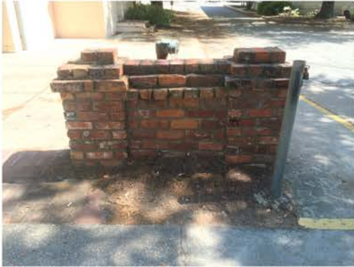
(196), Pendleton Street - Street Elevation Low wall height with piers.
