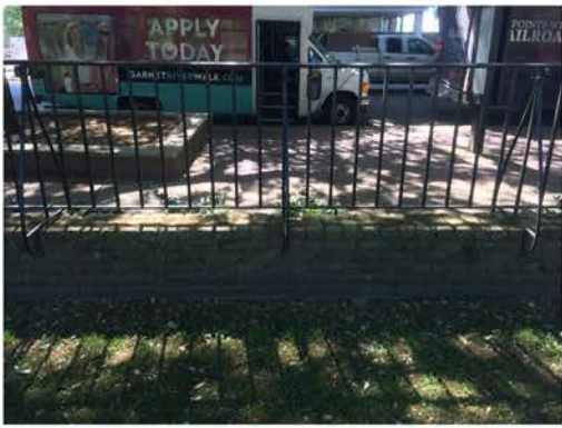
(229), Sumter Street - Campus Elevation Partial height wall with vertical rail. Vegetation issues typ.
