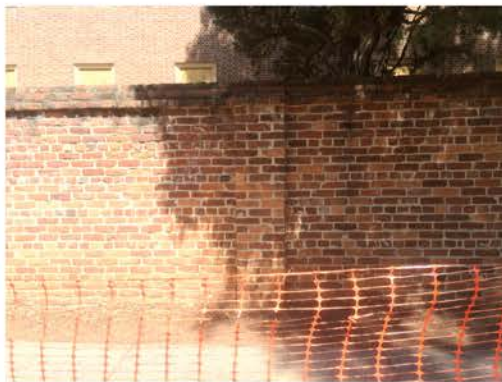
(59), Sumter Street - Street Elevation Full height wall with pier.
