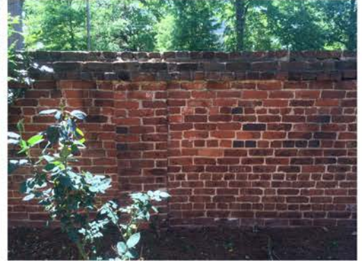
(90), Sumter Street - Campus Elevation Full height wall.
