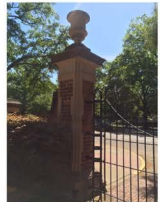
(96), Sumter Street - Campus Elevation Large Entry Pier with vertical rail and gate.
