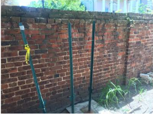
(4), Greene Street - Campus Elevation Full height wall.
