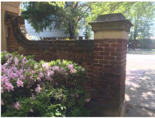
(241), Sumter Street - Campus Elevation Full height wall - two piers.
