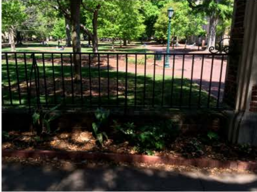
(100), Sumter Street - Street Elevation Partial height wall with vertical rail.
