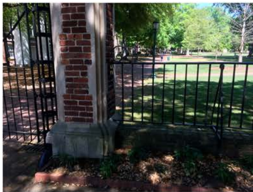
(119), Sumter Street - Street Elevation Partial height wall with large pier and gate.
