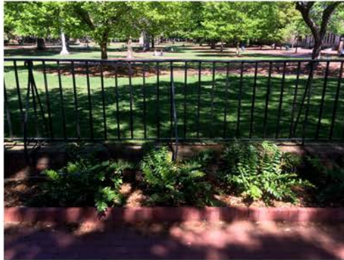
(104), Sumter Street - Street Elevation Partial height wall
