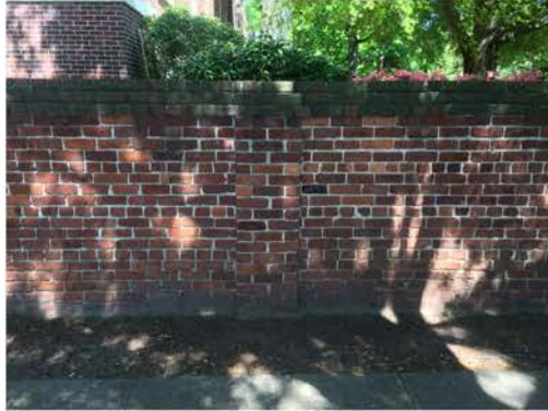
(125), Sumter Street - Street Elevation Full height wall. Cap repair.
