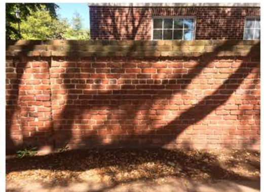
(132), Sumter Street - Street Elevation Full height wall with small pier.
