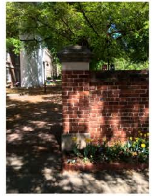
(123), Sumter Street - Street Elevation Full height wall with small pier. Signage.
