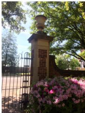
(239), Sumter Street - Campus Elevation Full height wall with vertical rail to large stone brick pier. Gate.
