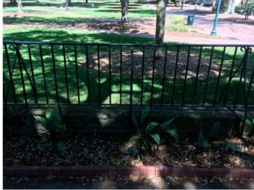
(101), Sumter Street - Street Elevation Partial height wall with vertical rail.
