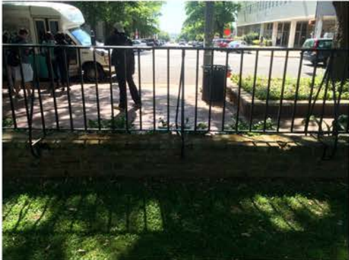
(220), Sumter Street - Campus Elevation Partial height wall with vertical rail. Vegetation issues typ.
