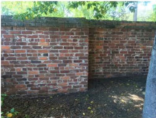
(19), Sumter Street - Campus Elevation Full height wall.
