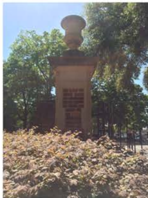
(95), Sumter Street - Campus Elevation Large Entry Pier with vertical rail and gate.
