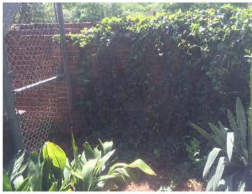
(86), Sumter Street - Campus Elevation Full height wall -new photo required.
