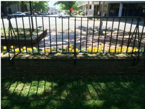
(223), Sumter Street - Campus Elevation Partial height wall with vertical rail. Vegetation issues typ.
