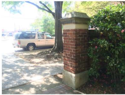
(242), Sumter Street - Campus Elevation Full height wall - single entry pier.
