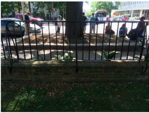
(217), Sumter Street - Campus Elevation Partial height wall with vertical rail.
